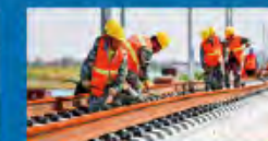
Railway track engineering
