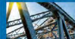
steel structure construction
